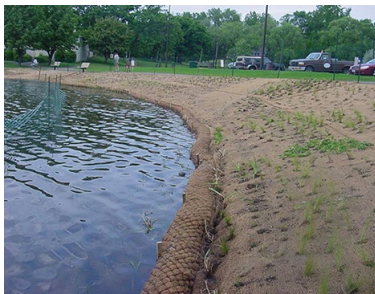
Coconut coir fiber logs providing a wave break for new plantings.
