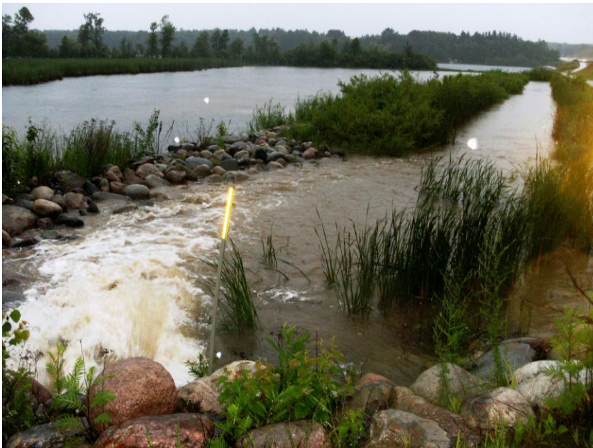
Figure 93: Highway 169 Pokegama causeway storm water retention pond after June 2012 storm event.
