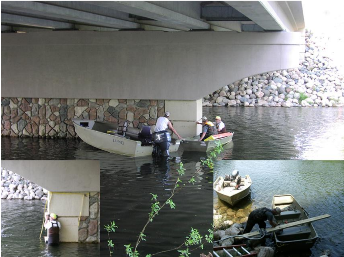
Figure 30: MPCA and ICSWCD install acoustic doppler current profiler on Pokegama outlet.
