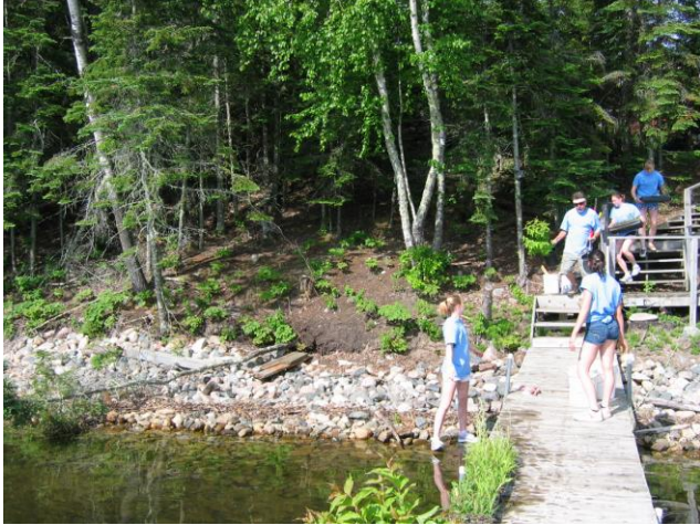
Images 4 and 5. Owner B property south (above) and north (right) of stairs before planting. Note: riprap previously installed to protect from wave/ice erosion at toe of slope. Erosion still occurring in sparsely vegetated upland area.
